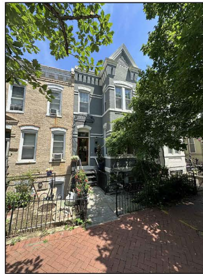
view from F Street NE from across the street
