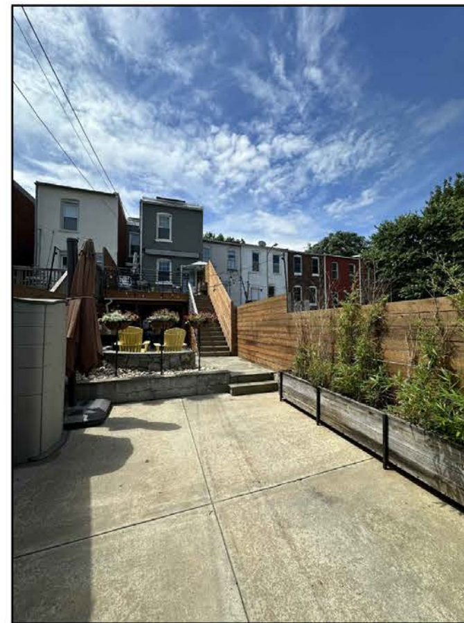
view of rear facade from parking pad
