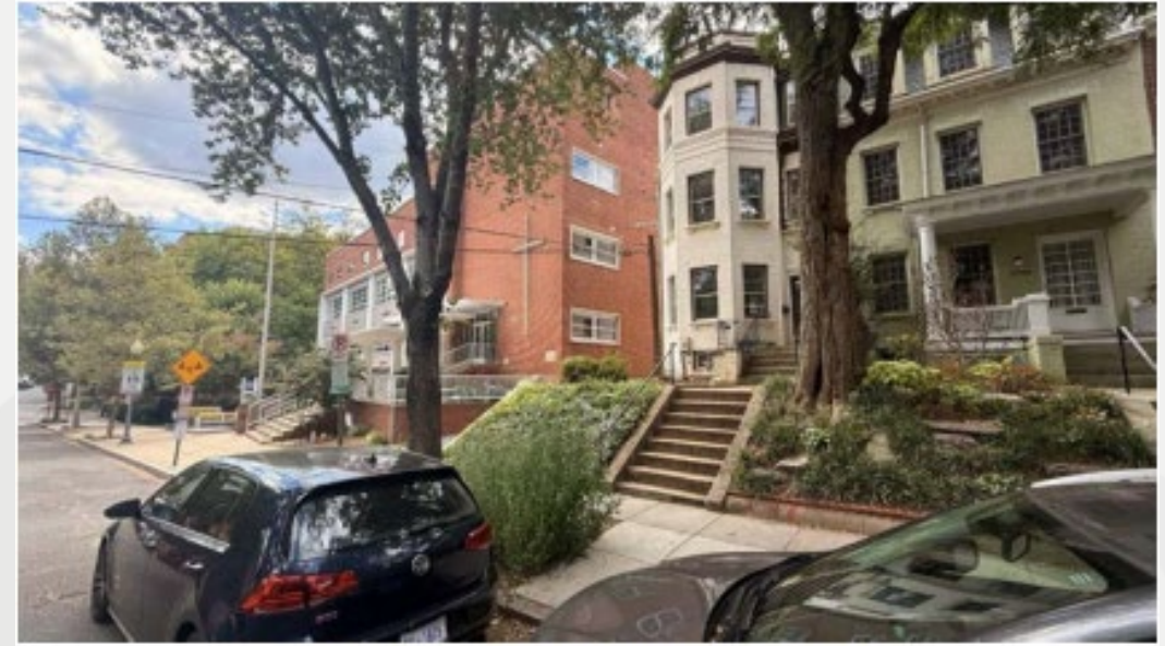
VIEW LOOKING SOUTH ALONG 27TH ST NW
