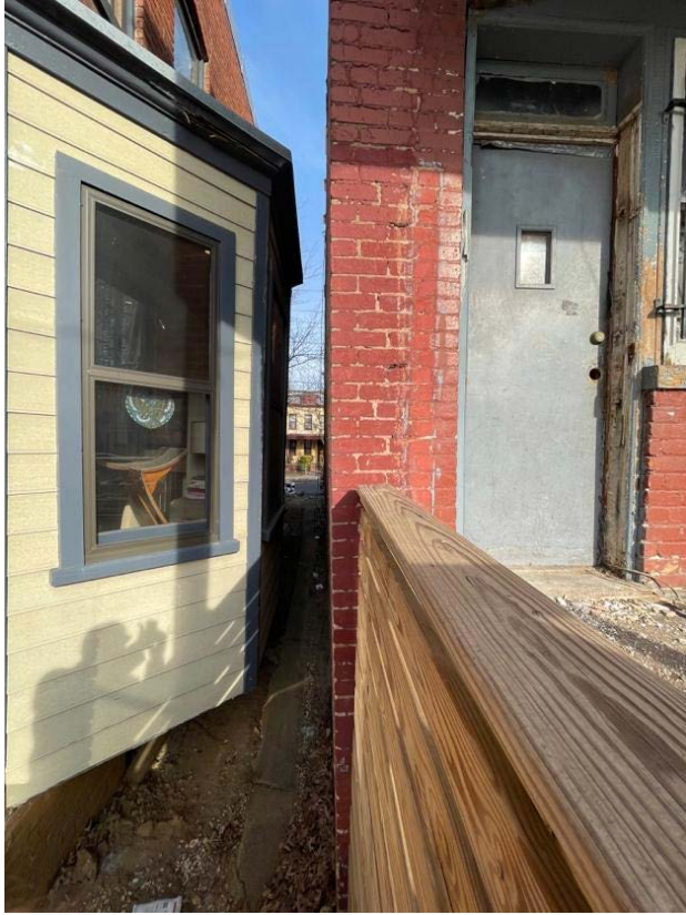
Property line between 934 Shepherd Street (left) and the Property (right), showing the proximity of the proposed construction to the neighboring wall and window – 18 inches.
