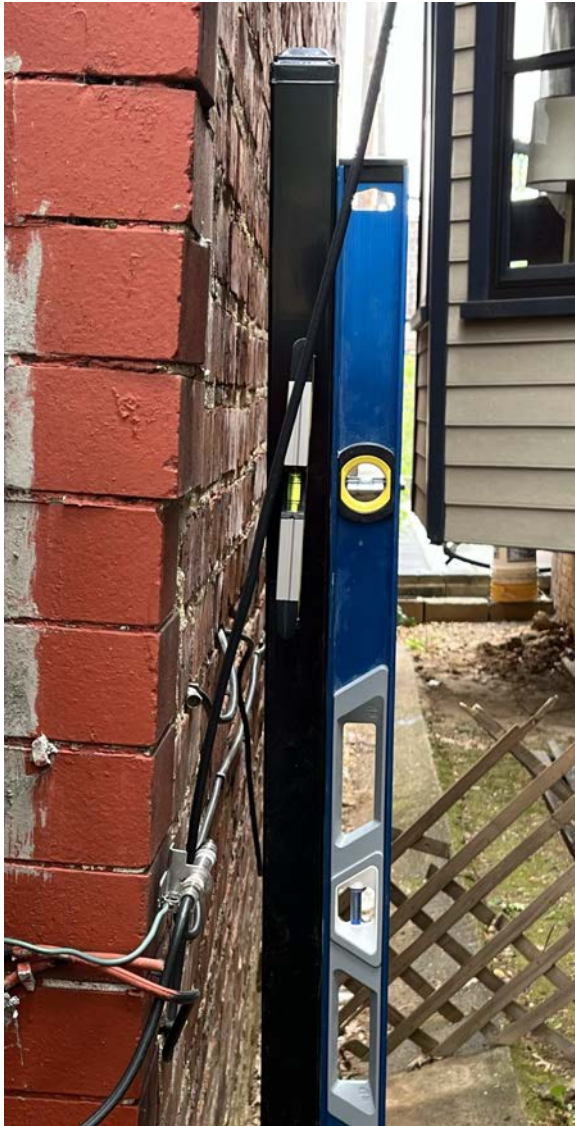
A level held against gate post documenting 932 Shepherd Street western wall's lean toward 934 Shepherd Street.
