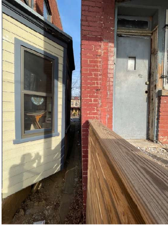
Property line between 934 Shepherd Street (left) and the Property (right).
