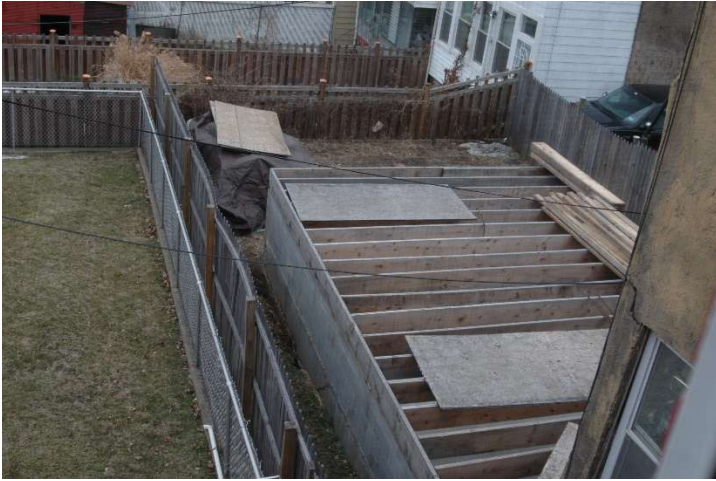
February 2011 – second addition foundation poured and walls constructed
