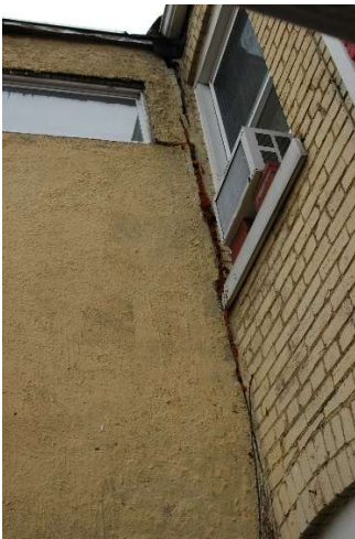
2011- first addition separating from house
