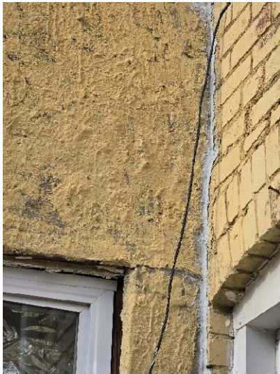
Jan 2026 – filler in the crack between the first addition and the house
