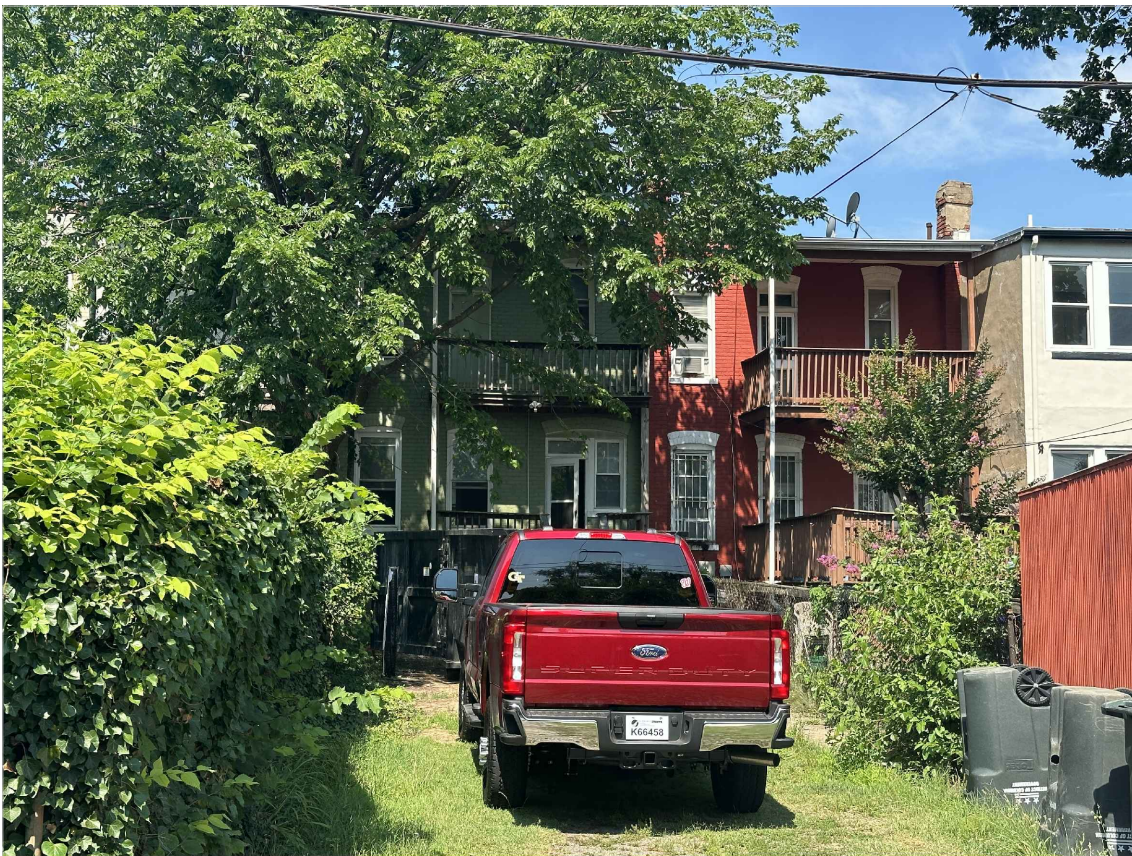
view of rear facade from alley
