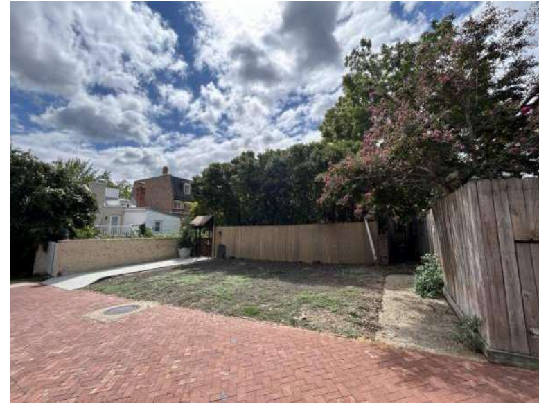
VIEW OF PROPERTY FROM PROSPECT STREET
