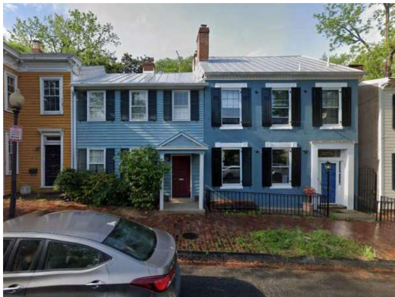
VIEW OF BUILDINGS ACROSS THE STREET
