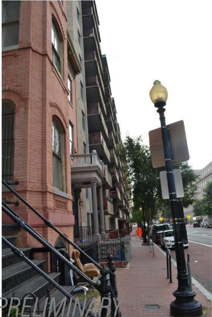
3 EXISTING SIDEWALK VIEW SCALE: NONE
