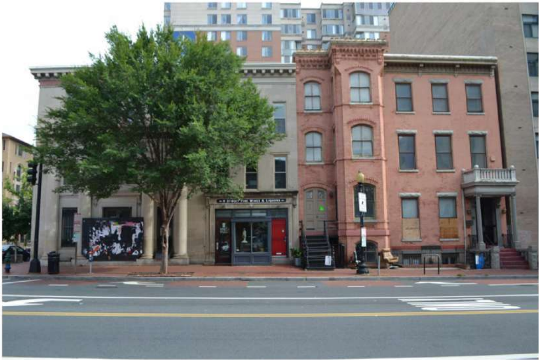
2 EXISTING FRONT VIEW SCALE: NONE
