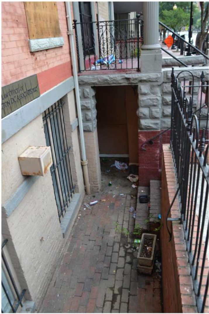
5 EXISTING WALKWAY VIEW SCALE: NONE
