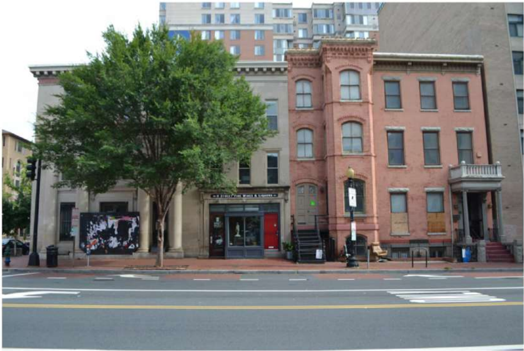
2 EXISTING FRONT VIEW SCALE: NONE
