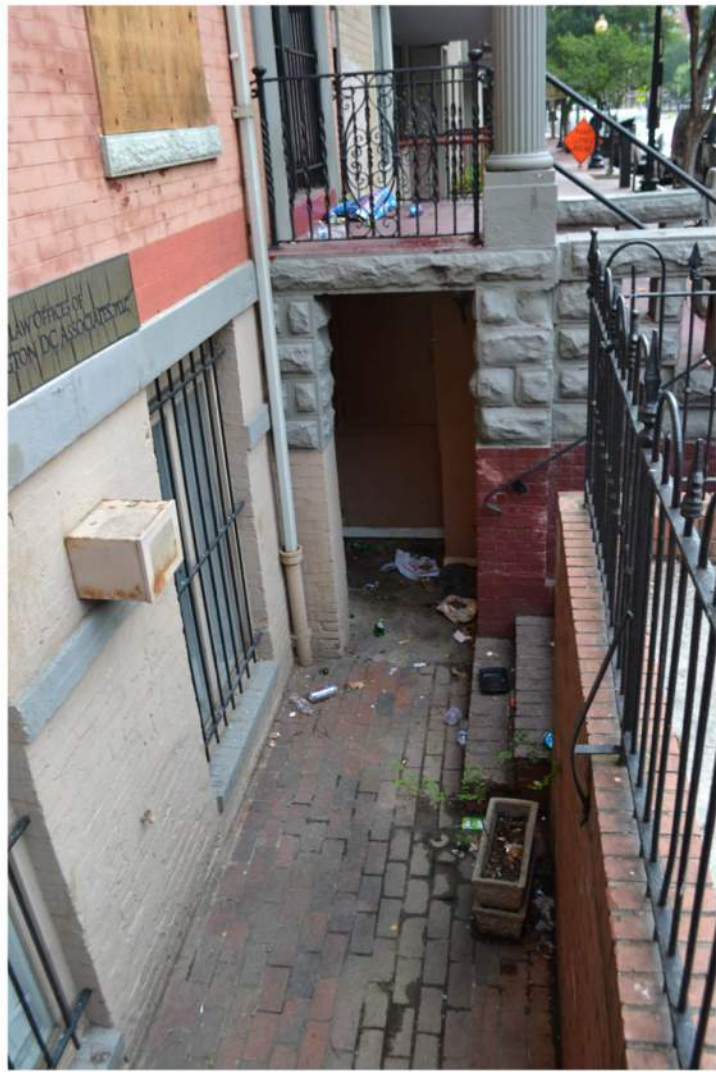
5 EXISTING WALKWAY VIEW SCALE: NONE
