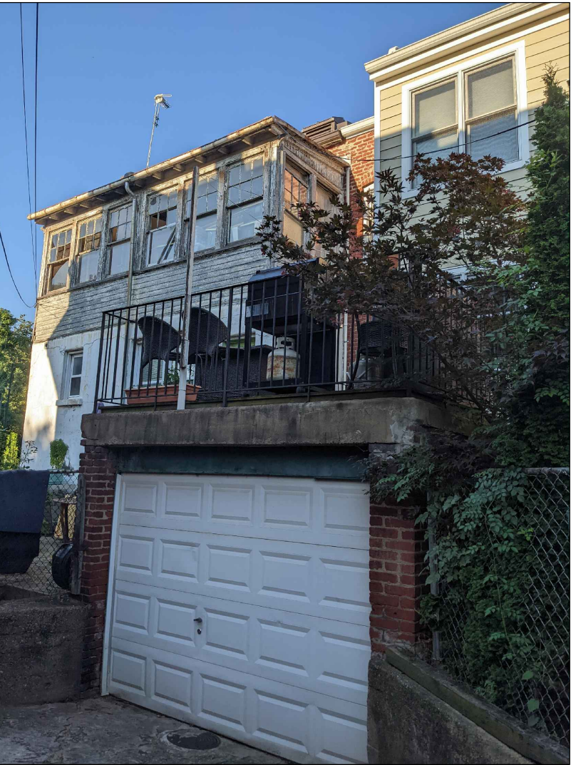
424 7TH ST NE - IMAGE FROM REAR ALLEY, 422 7TH ST NE GARAGE AT FRONT
