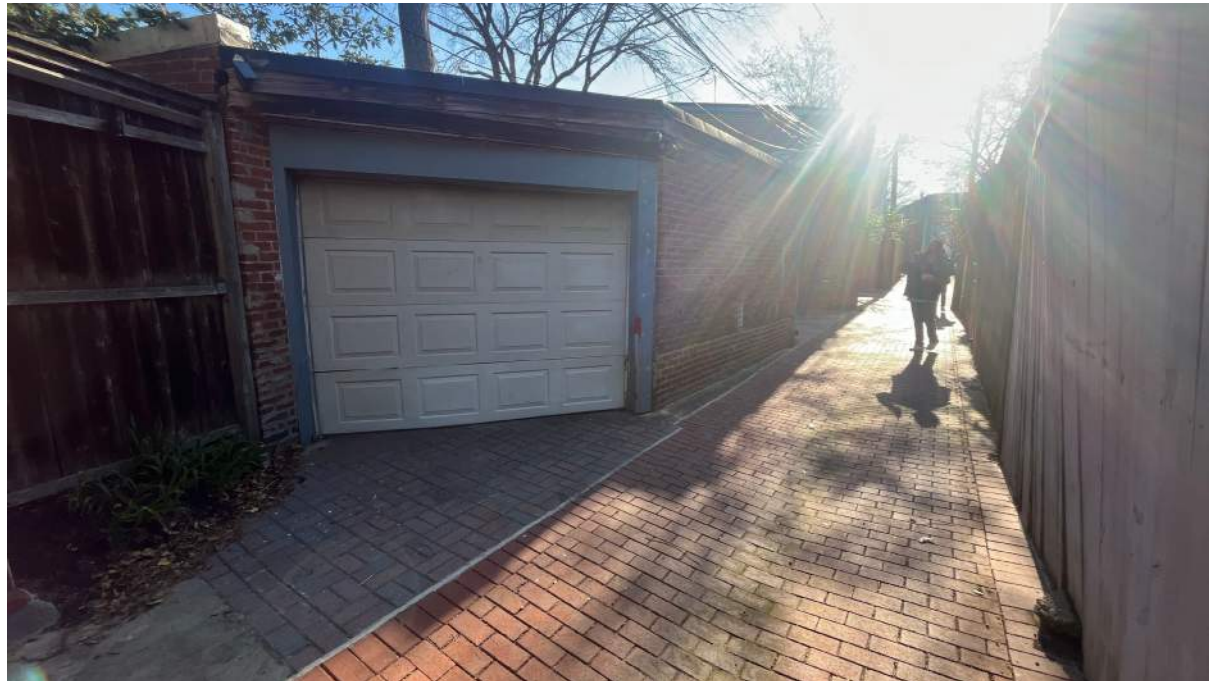
1. VIEW LOOKING ALLEY LOOKING EAST
