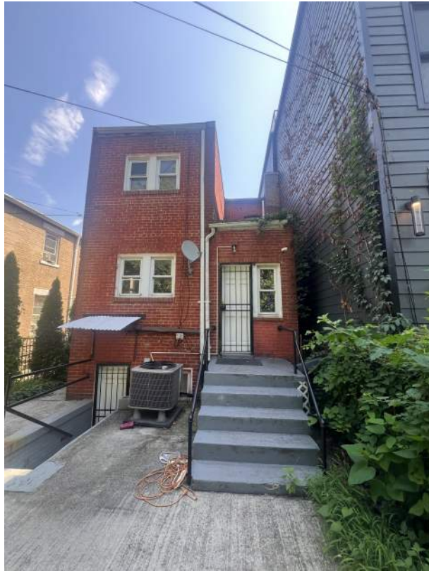
1. WEST(REAR) FAÇADE OF SUBJECT PROPERTY FROM THE REAR YARD.
