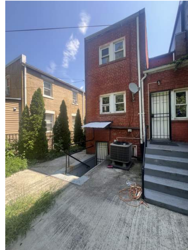
2. VIEW TOWARDS 2712 SHERMAN AVE NW FROM REAR YARD OF PROPERTY.
