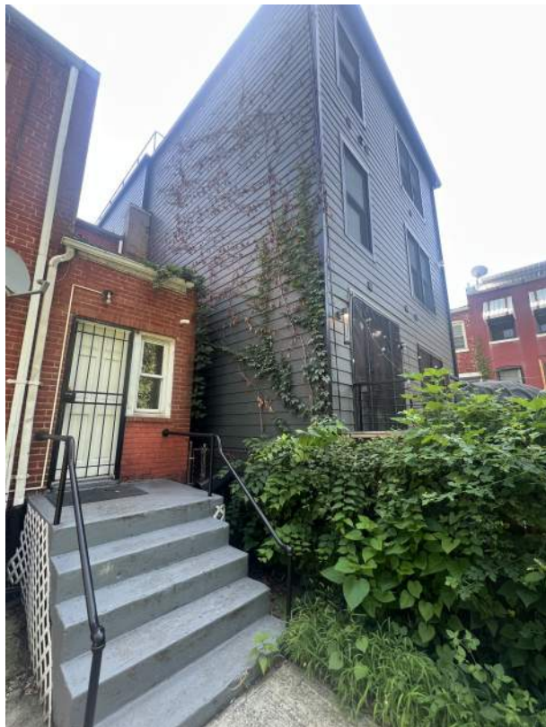
3. VIEW OF 2708 SHERMAN AVE NW FROM REAR OF SUBJECT PROPERTY.
