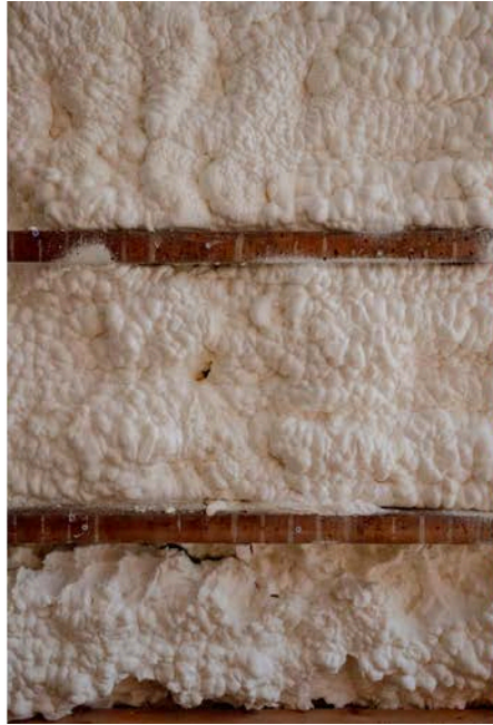
Left: Aramis Rosa used passive design elements to renovate his family's new home. Center: Spray foam insulation in the house's walls cuts down on heating and cooling costs. Right: Rosa did most of the remodeling himself.
