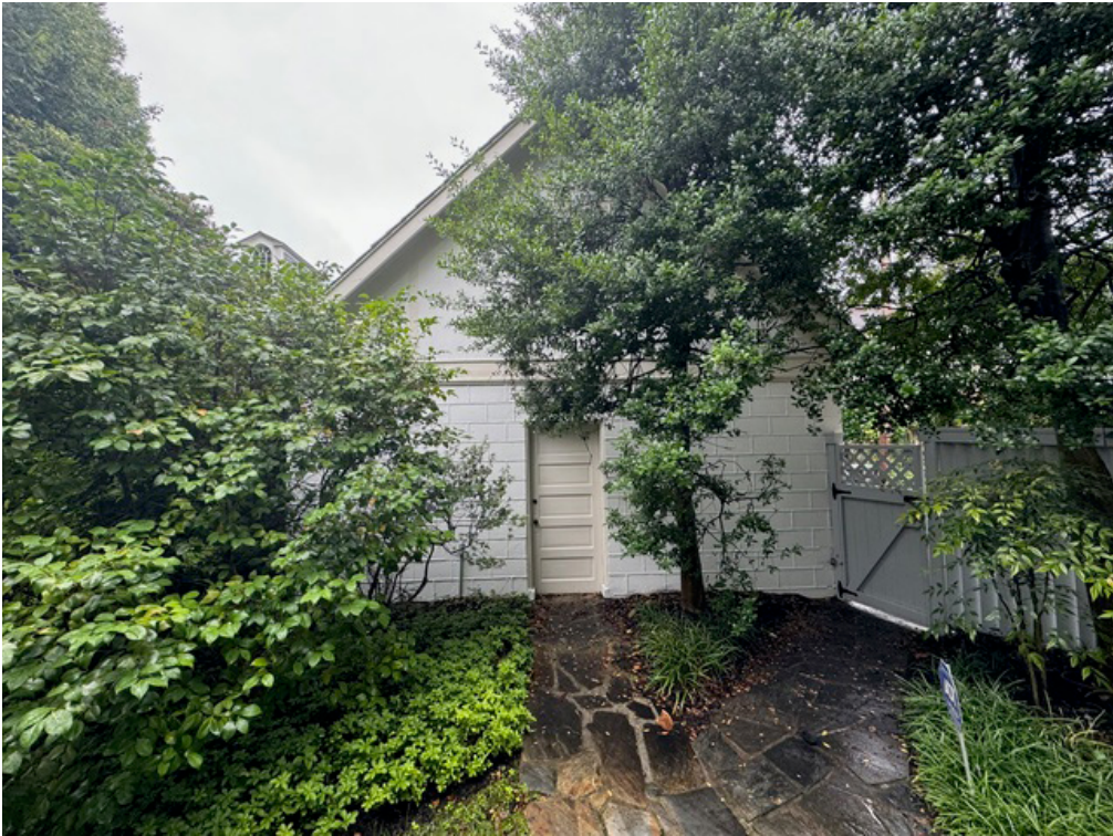
4. Rear- Looking south at the existing garage
