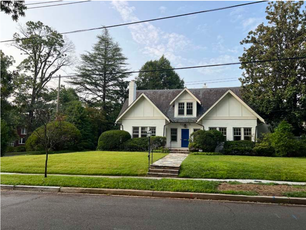
1. Front- Looking south
