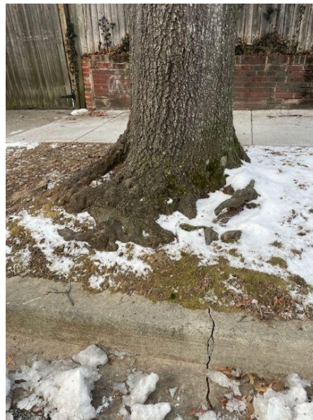
23" Scarlet oak. Notice cracking curb, recently repaired sidewalk, retaining wall, girdling roots and mounded root flares.
