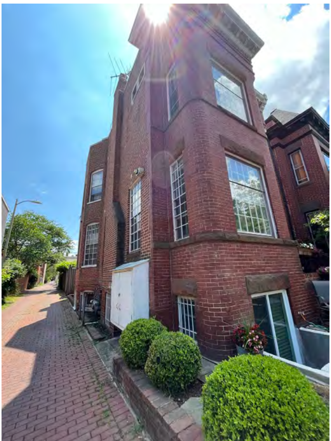
VIEW DOWN ALLEY FROM A STREET NE
