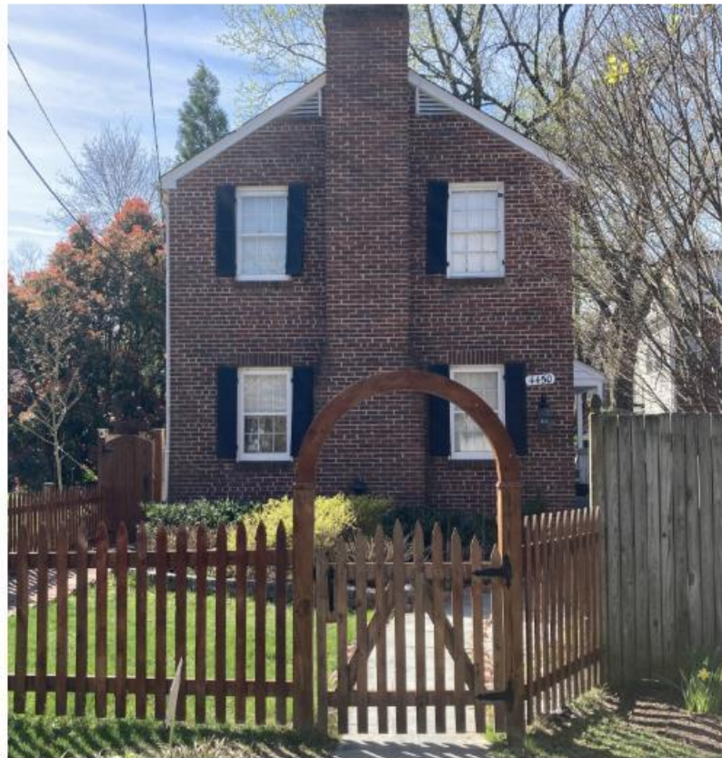
STREET FRONTAGE - NORTH FACADE
