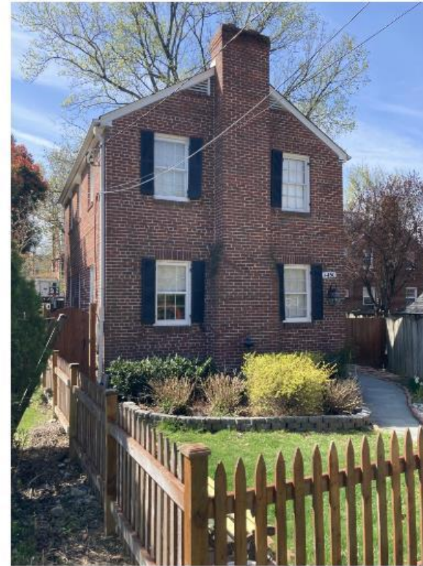
EAST SIDE YARD FROM STREET
