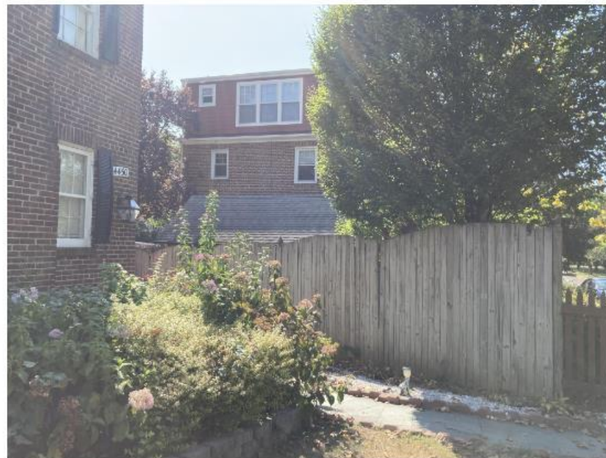
LOOKING WEST TO ADJACENT PROPERTY
