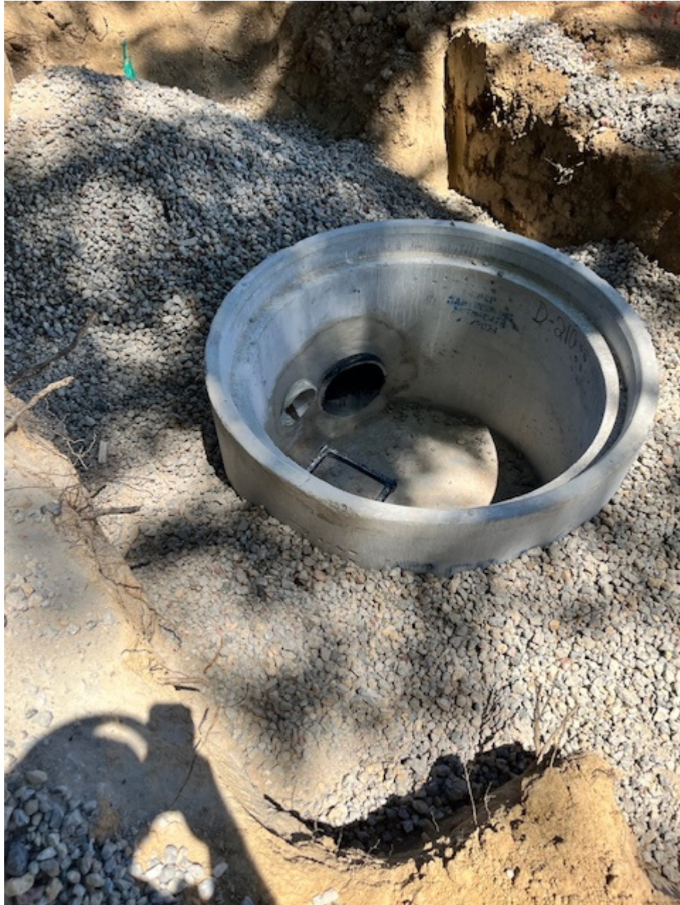
Figure 6: SWM utility work backfilling
