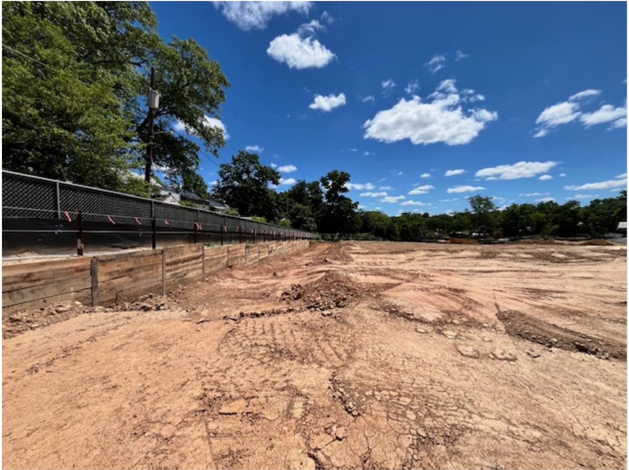
Figure 3: Earthwork for retaining wall (Northwest).
