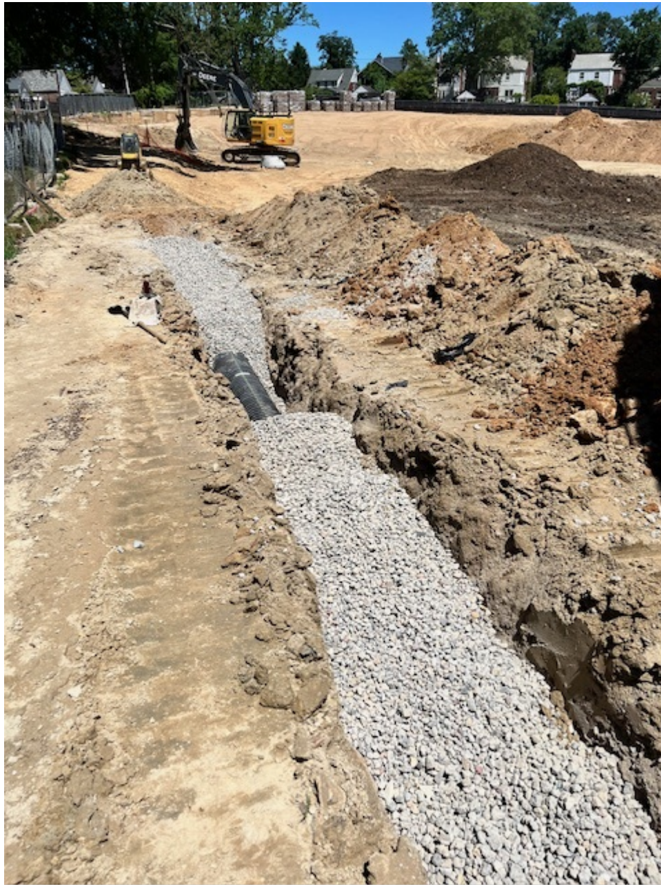
Figure 4: Stormwater Management Structures
