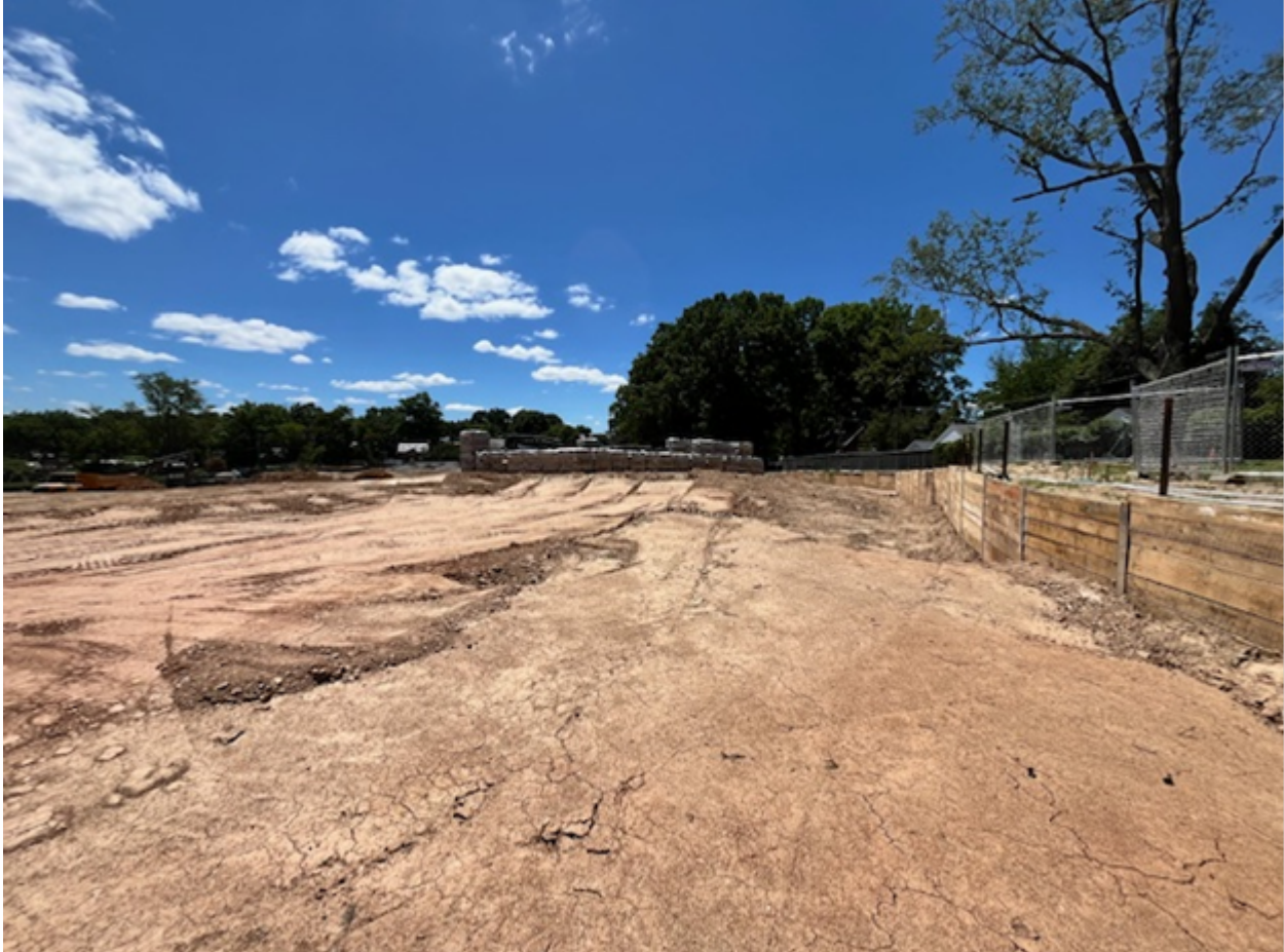
Figure 2: Earthwork for retaining wall (Northwest).
