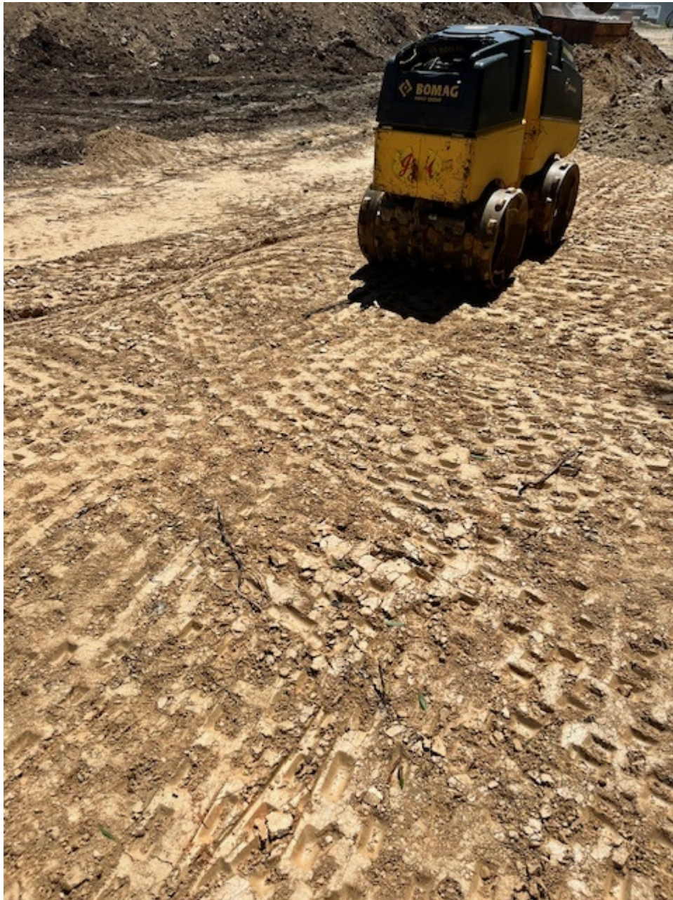
Figure 5: SWM utility compaction
