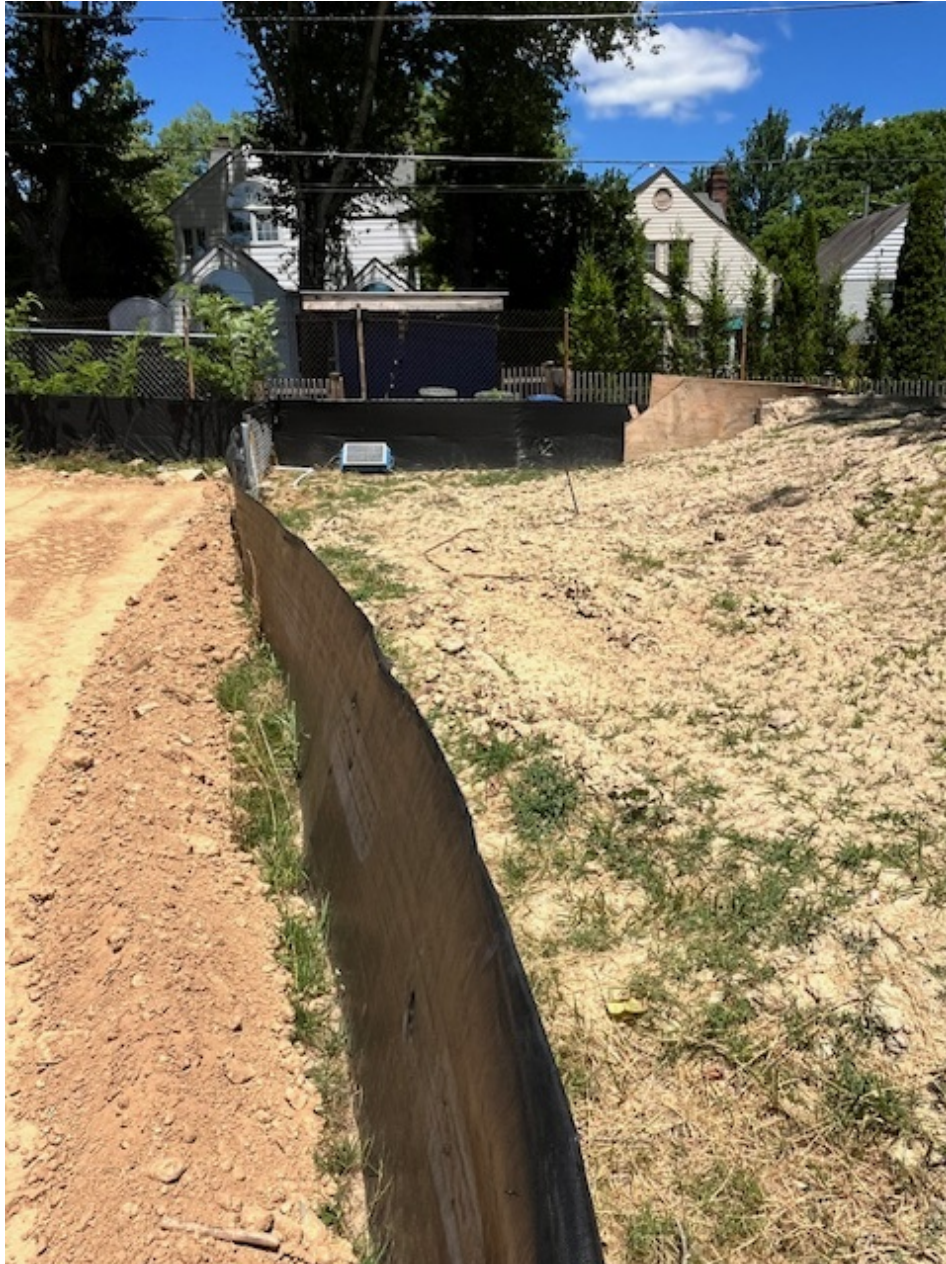
Figure 9: Vibration Monitoring – UM16648
