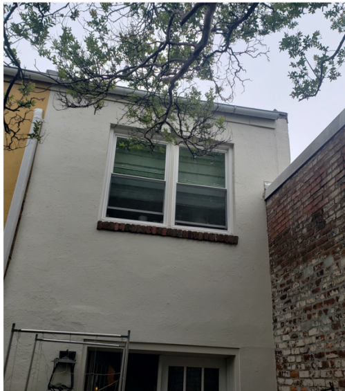
Photo of bedroom windows (left) and bathroom window (right) of 520 Archibald Walk SE in close proximity to the roof of #633. Also depicts integration of 520's western wall into the eastern wall of 633. Rear E Street SE, illustrating how the wall of 520 is integral to the structure of 633.
