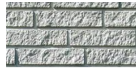
BRICK PATTERN ON CONCRETE FOUNDATION WALLS
