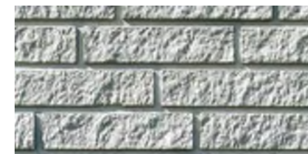
BRICK PATTERN ON CONCRETE FOUNDATION WALLS
