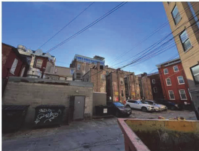
11. View of 507-511 H Street alley structures
