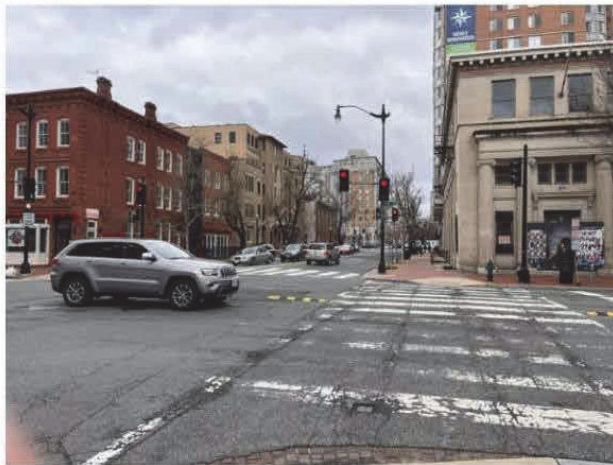
3. Looking North on 5th Street NW
