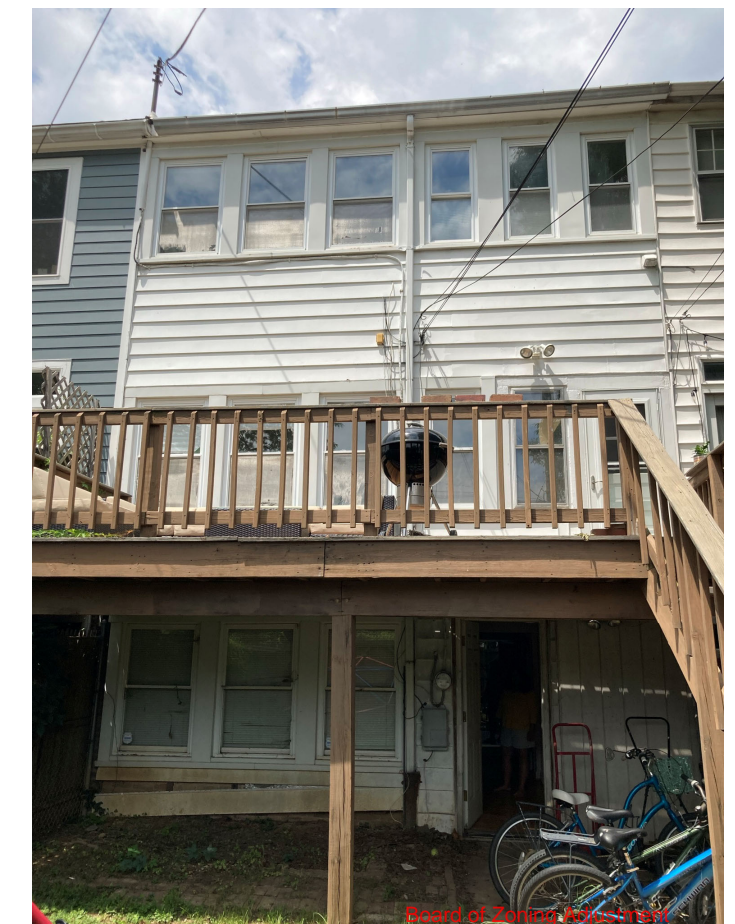
EXISTING REAR FACADE
