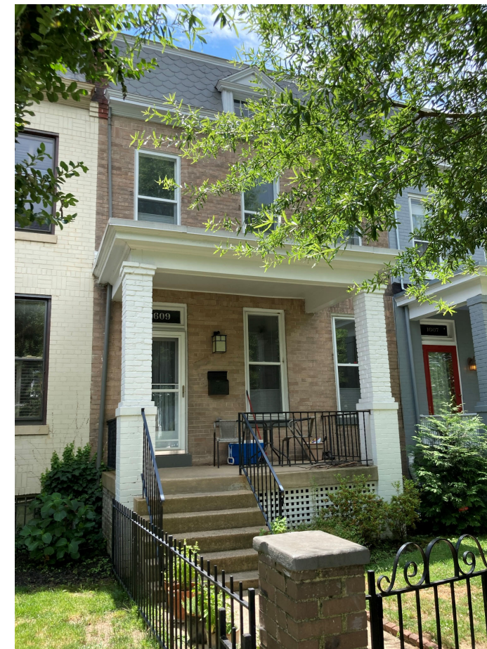
EXISTING FRONT FACADE
