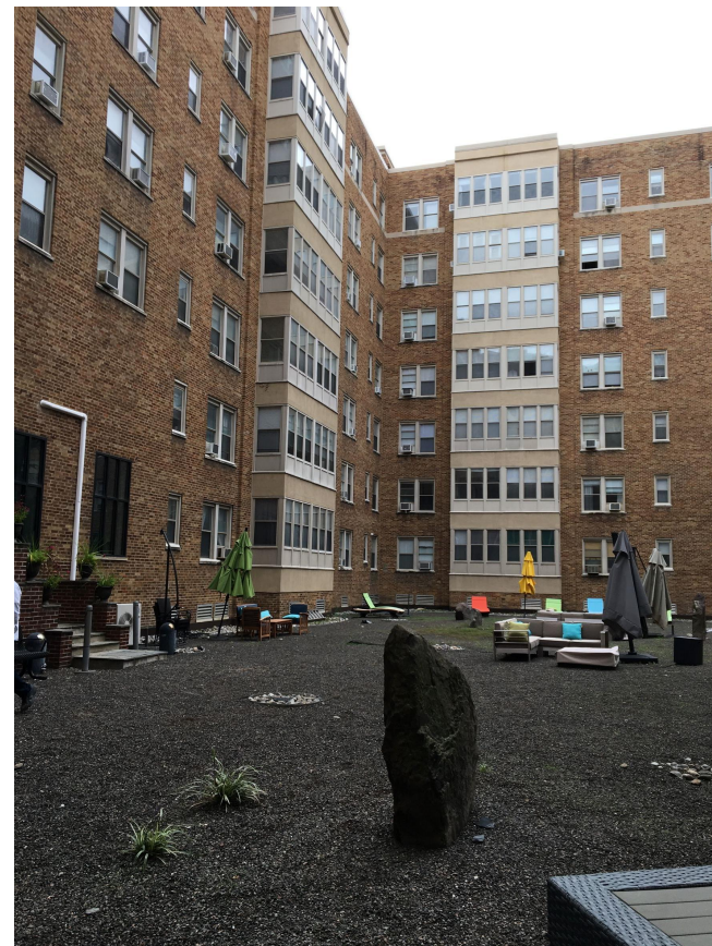
D - INTERIOR COURTYARD
