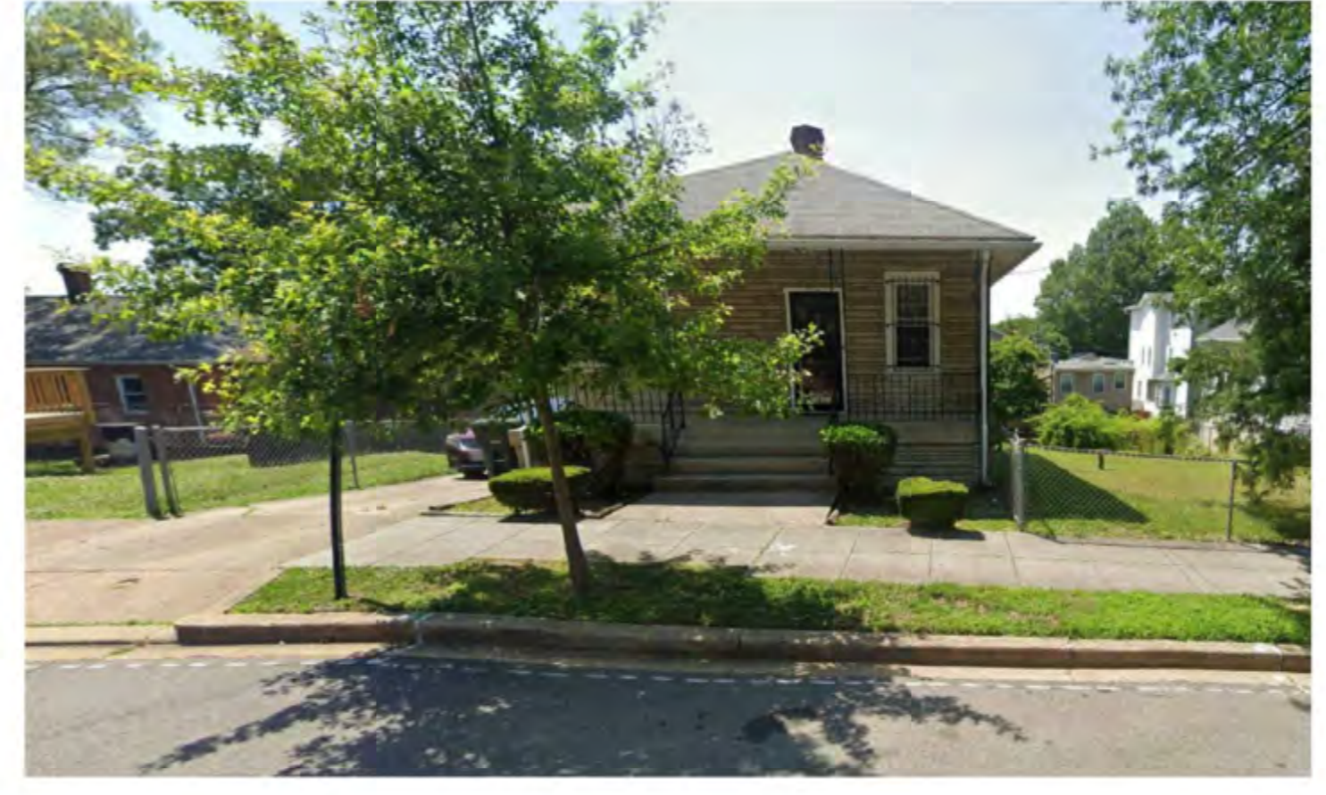
VIEW FROM 57TH STREET
