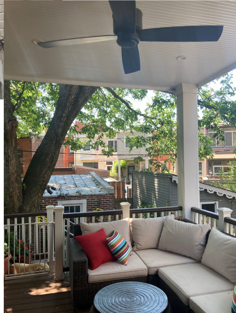
EXISTING 1ST FLOOR PORCH
