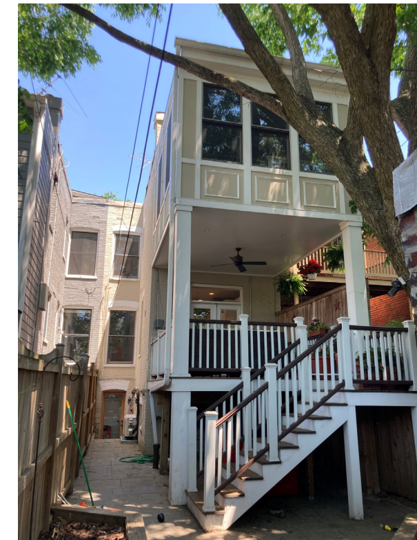
EXISTING REAR FACADE
