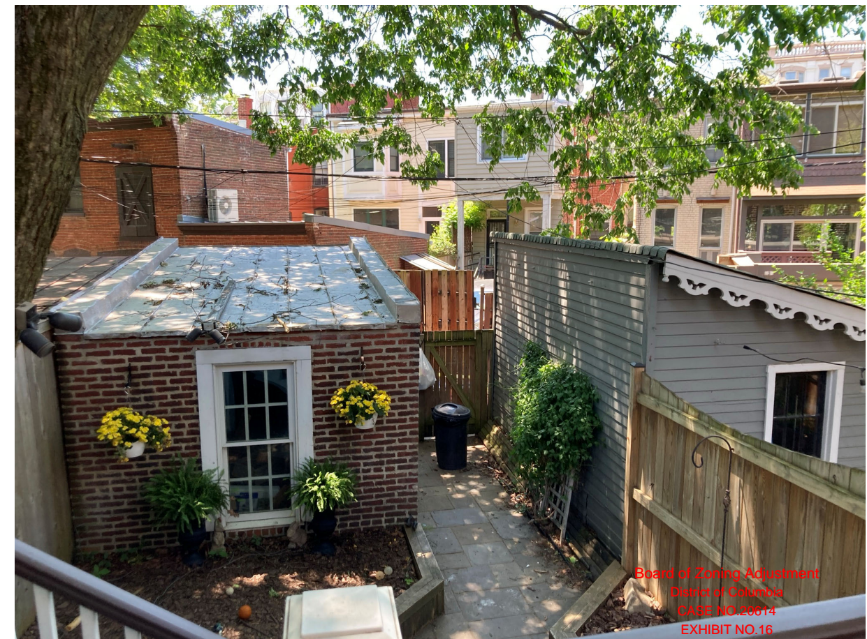
EXISTING REAR YARD
