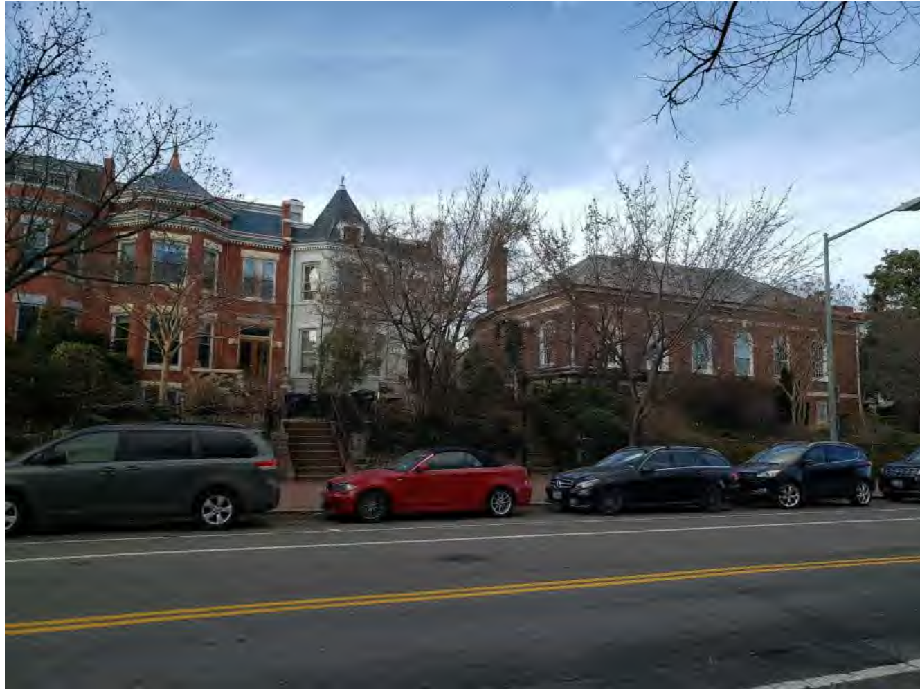
PHOTO - VIEW FROM SOUTH CAROLINA AVE.
