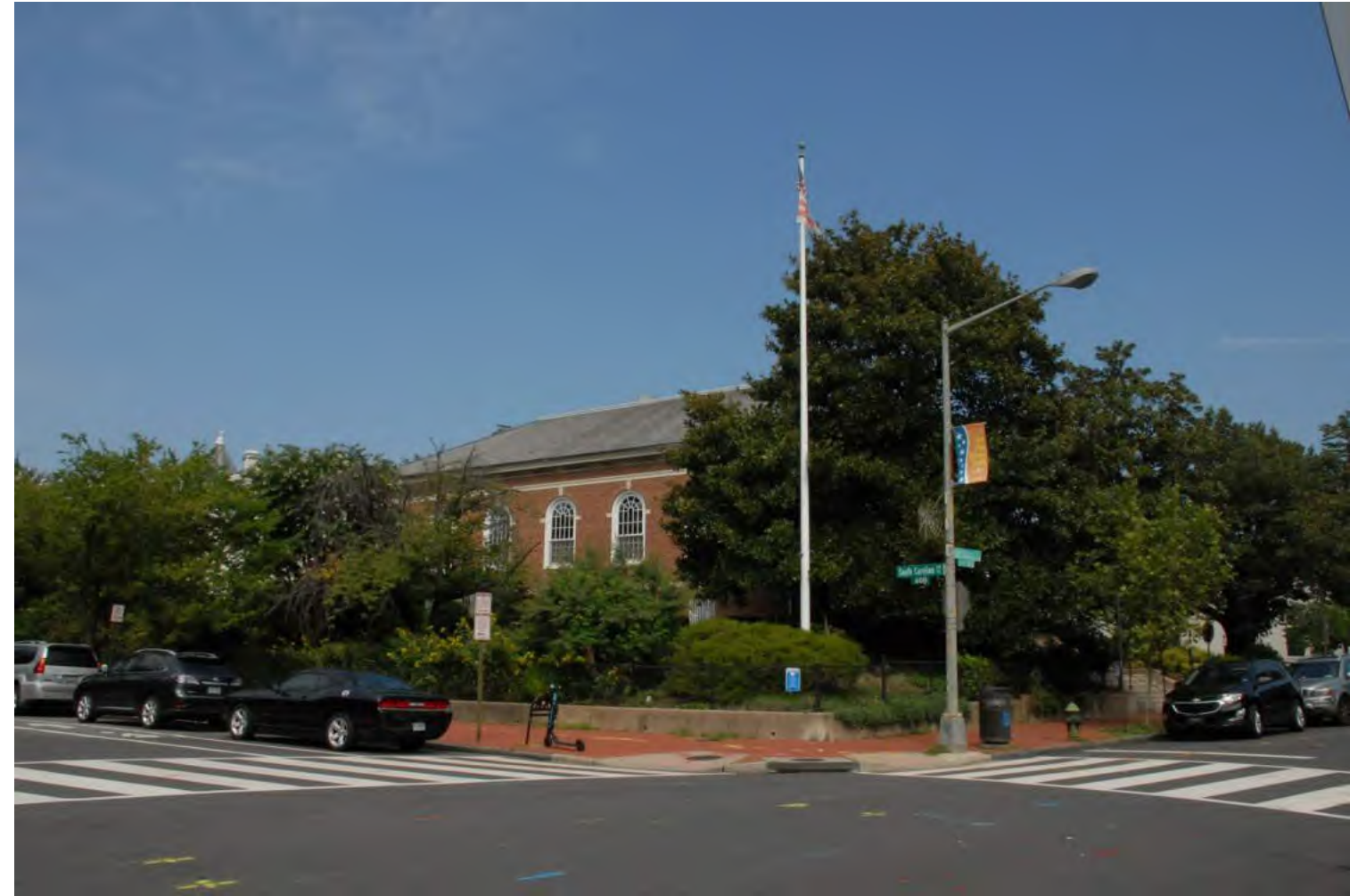
PHOTO - VIEW FROM CORNER OF SOUTH CAROLINA AVE. AND 7TH ST.
