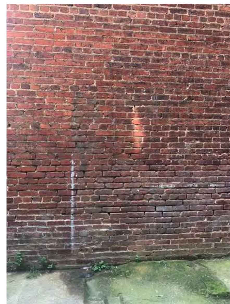
NEIGHBORS WALL ON OUR EAST PROPERTY LINE
