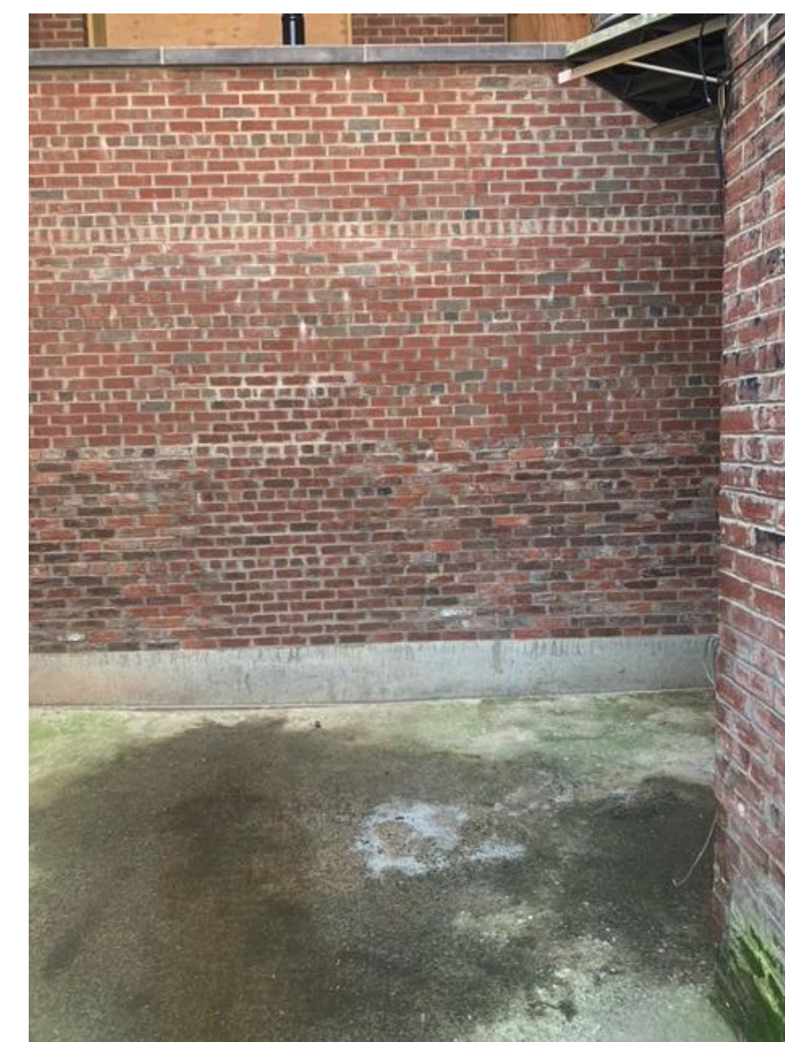
SOUTH PROPERTY LINE AT NEW DEVELOPMENT WALL
