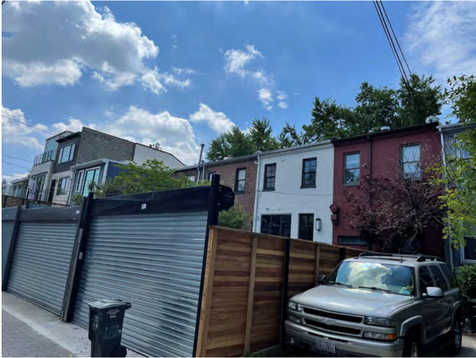
VIEW FROM ALLEY BEHIND JACOB'S LOOKING SOUTHEAST
