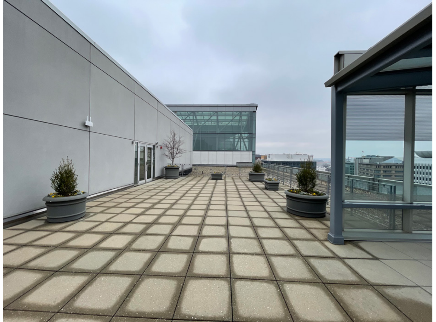
EXISTING PENTHOUSE SOUTH ELEVATION WITH EXISTING EMBELLISHMENT (RIGHT SIDE OF IMAGE) (1875 PENNSYLVANIA AVENUE NW BEYOND)
