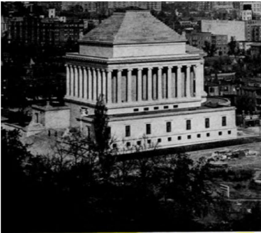
View of Building, Showing Solid Limestone Roof
