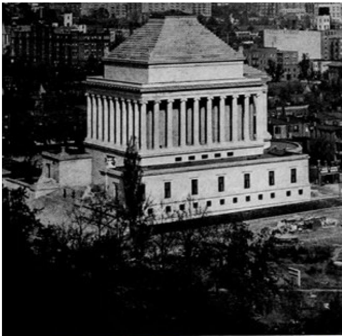
View of Building, Showing Solid Limestone Roof
