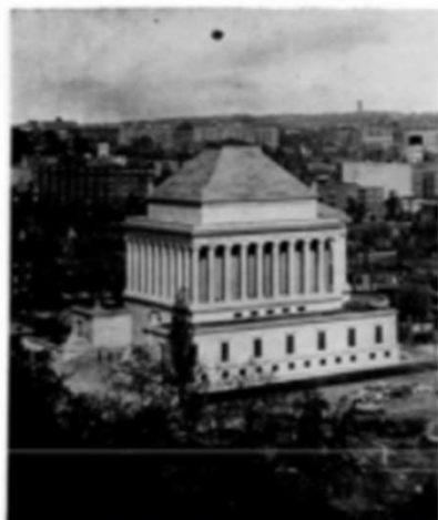
View of Building, Showing Solid Limestone Roof
