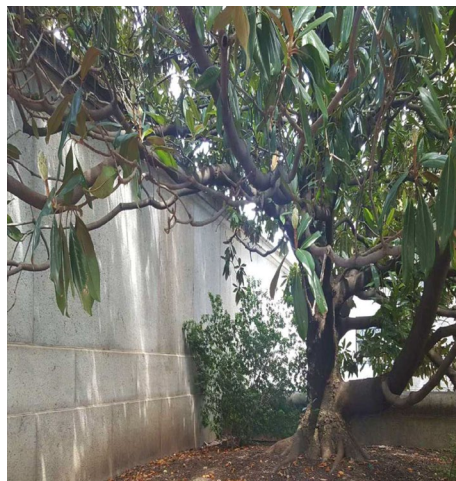
Photo 1 East Side of 11'6" Wall
