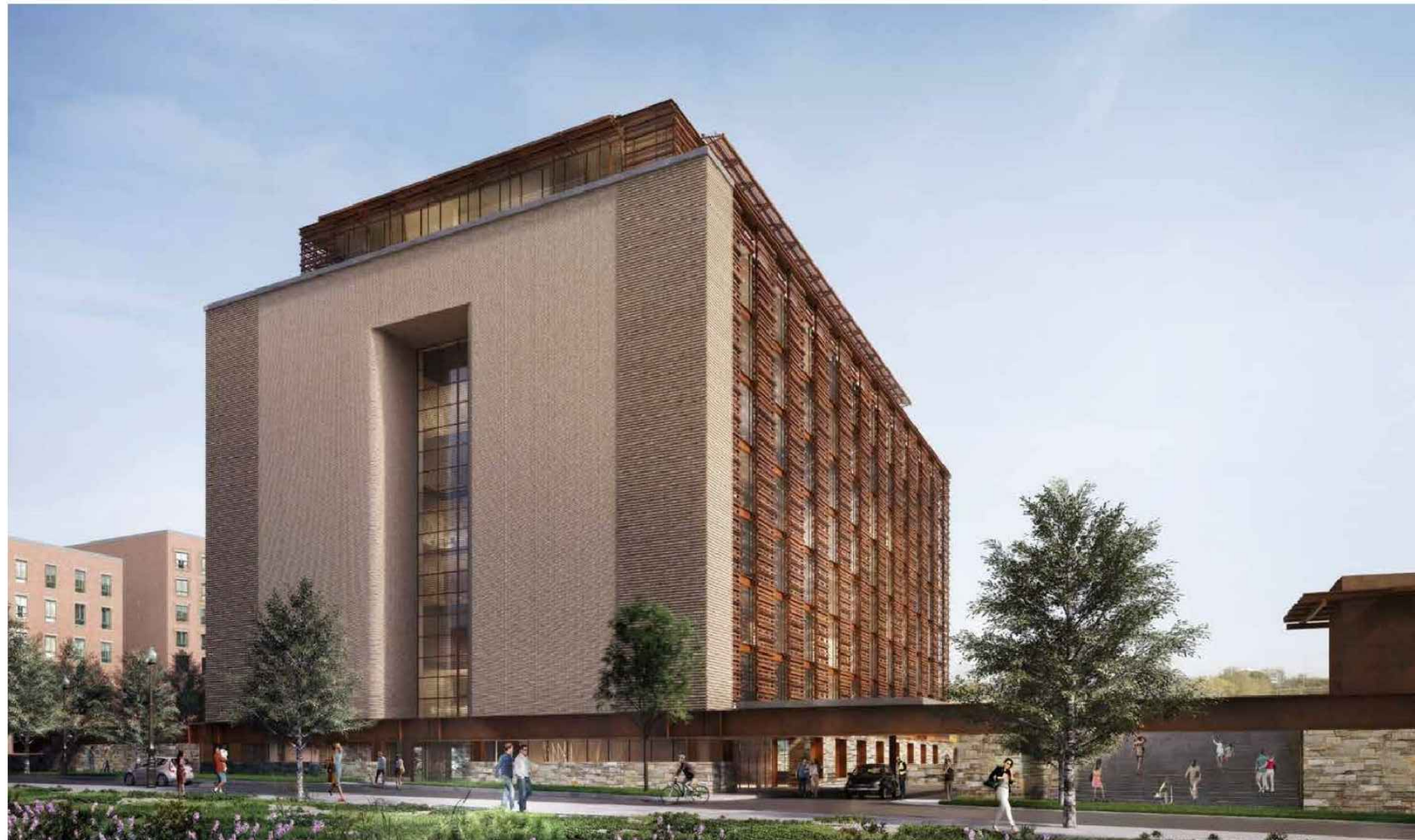
29TH STREET VIEW - OPEN PANELS
