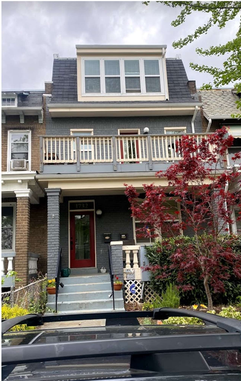
1732 Bay Street SE
