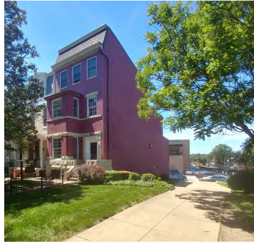
site and adjacent rowhouse
