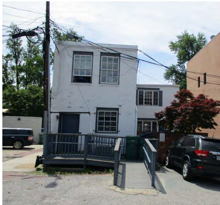
structure in alley to south
