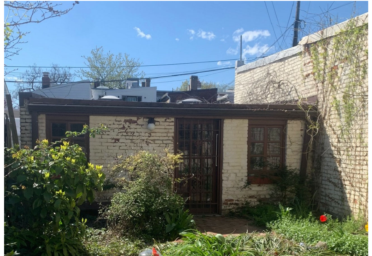
EXISTING GARAGE FROM BACK YARD
