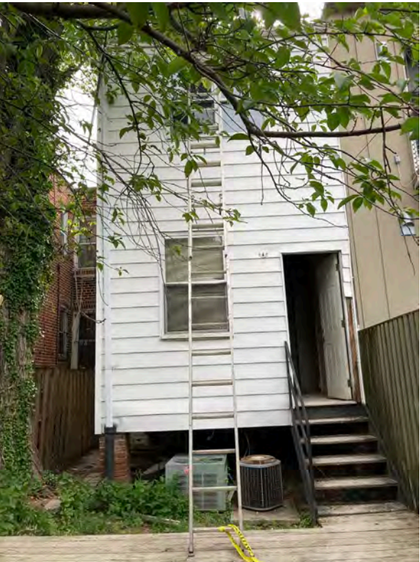
EXISTING REAR FACADE
