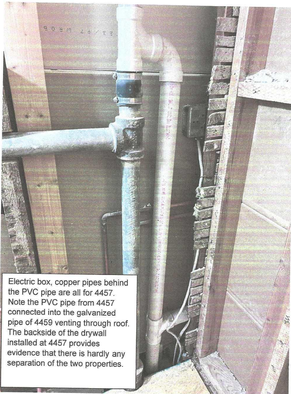
Figure 1 Electric, plumbing, vent inside the common wall 4457-4459
