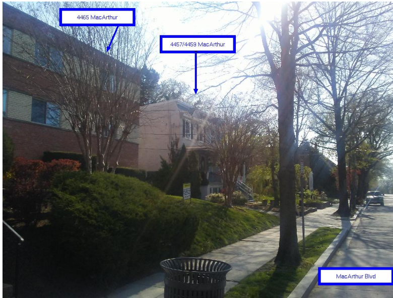
(a) 4457/4459 MacArthur Blvd, current view, 2021-04-08
