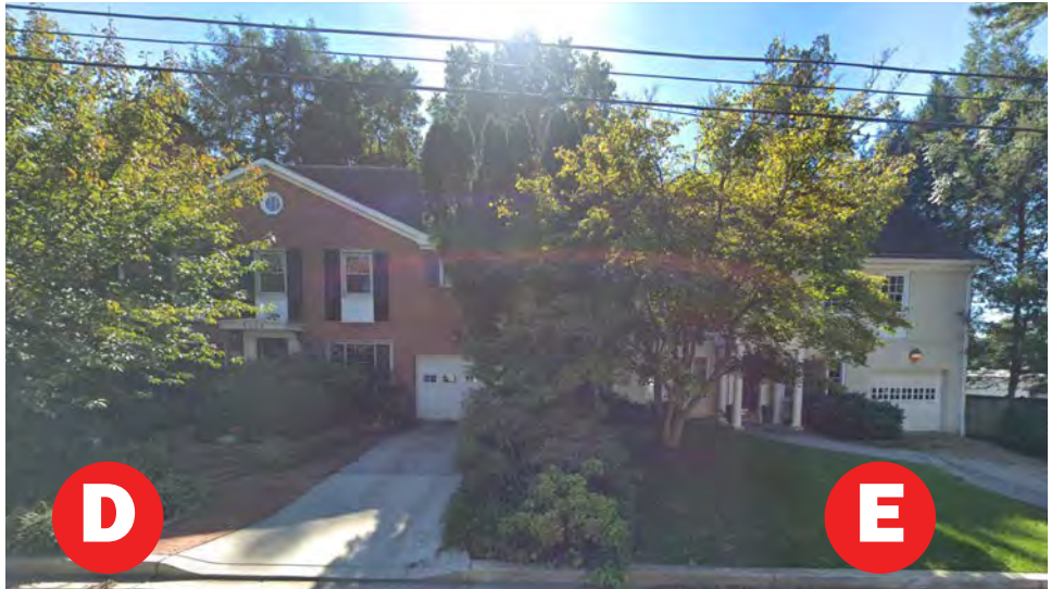
4808 V STREET NW (D-LEFT) & 4812 V STREET NW (E-RIGHT)
