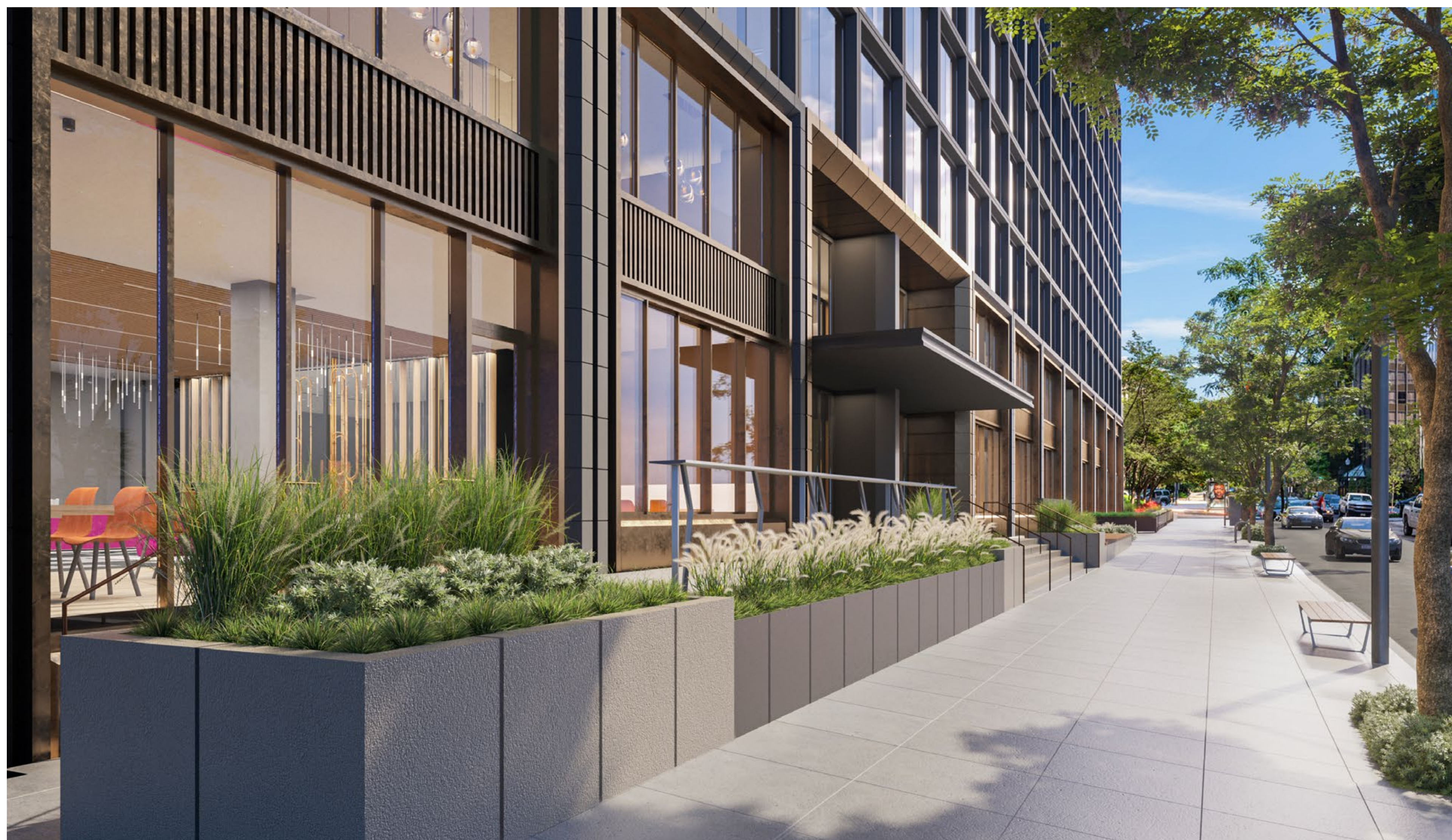
(1) VIEW LOOKING NORTH ON 21ST STREET
