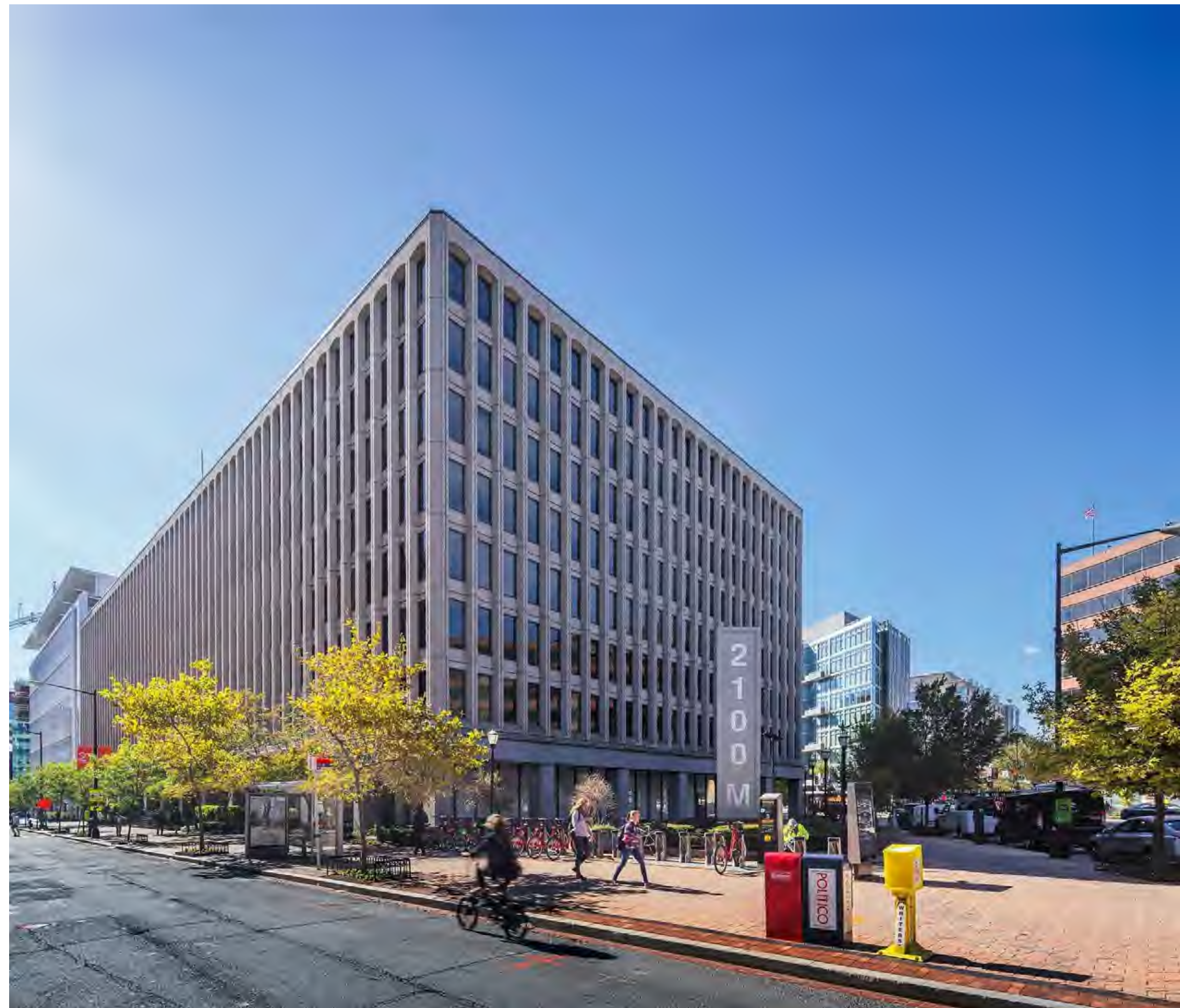
(3) VIEW FROM 21ST STREET CORNER
