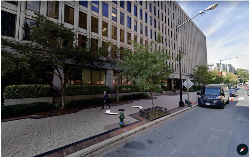
(4) VIEW FROM 21ST STREET
