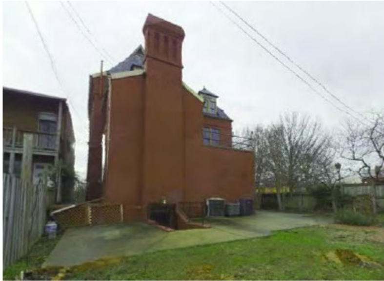
REAR YARD LOOKING SOUTHWEST
