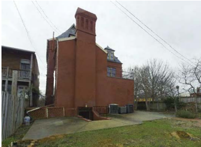
REAR YARD LOOKING SOUTHWEST
