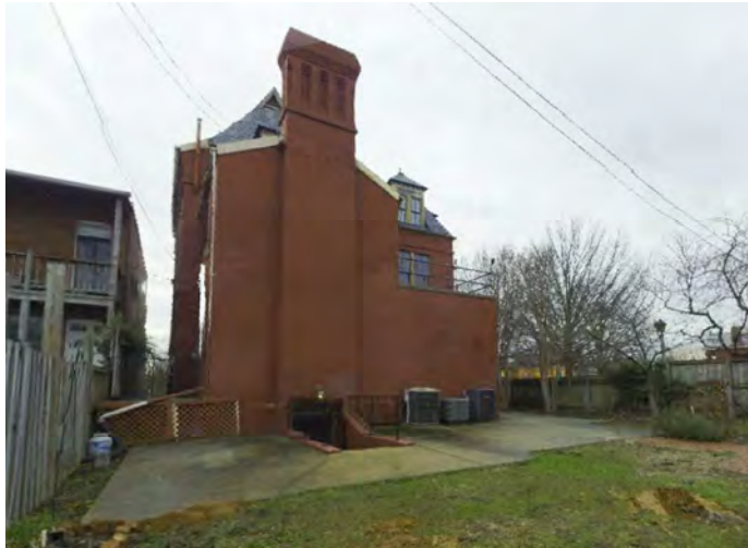
REAR YARD LOOKING SOUTHWEST
